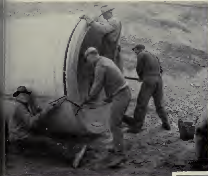
BER GASKETS on the spigot ends of the 20-foot concrete sections of the big water pipe made it water-tight (see above). At the right, columns supporting the Terminal Reservoir roof. At the bottom, covering Terminal Reservoir No. 2 with a slab roof.
